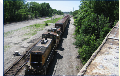
Existing conditions P2 project
