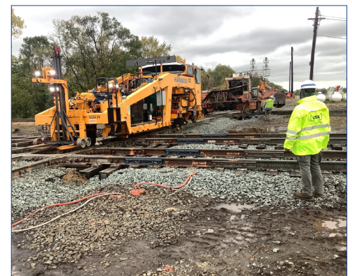
Construction team doing track work at the Forest Hill (P3) site.
