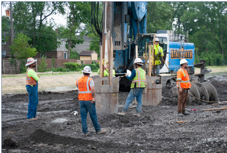
Construction team drilling shafts for the Forest Hill Flyover (P3) Project.
